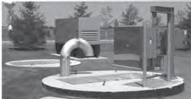
Lift Stations-New and Retro-fit Upgrades
