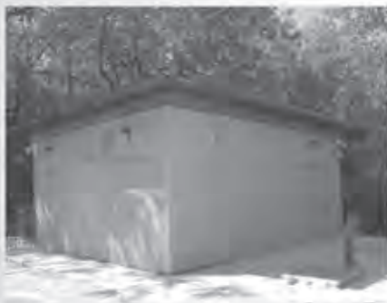
Housed Pump Systems
